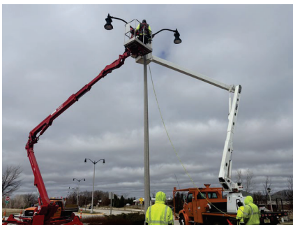
Figure 2-STH33 Light pole relocation
