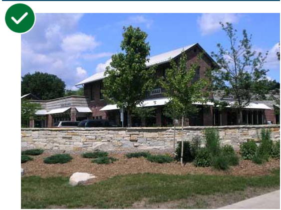
Exhibit 22-7. An example of a masonry wall shielding the parking area for a retail center
