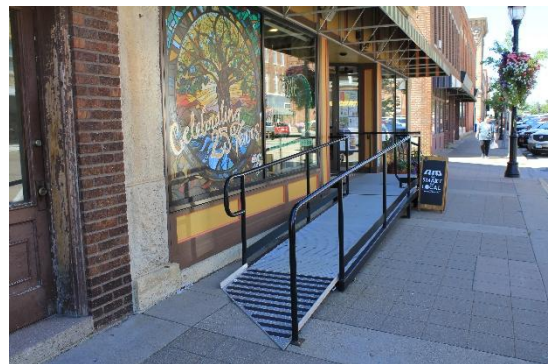
Exhibit 21-3. An example of an encroachment in a public sidewalk
